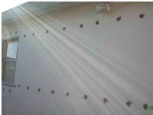
Typical Wall Drilling – 2 holes per bay
